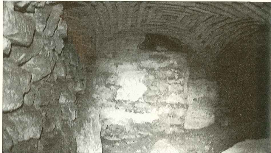
Fig. 45 - The Room Under the Northwest Ramp.
