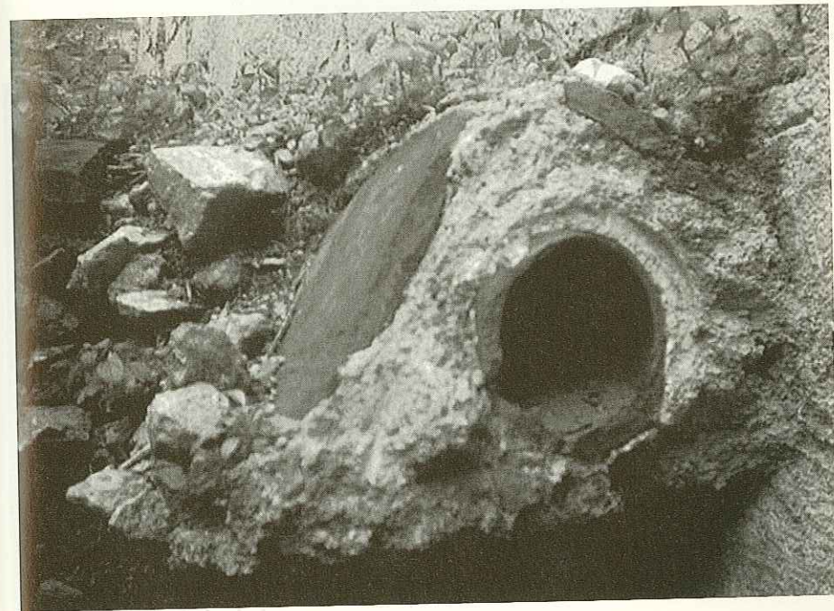
Fig. 17 - The teracotta pipes in the western courtyard.
